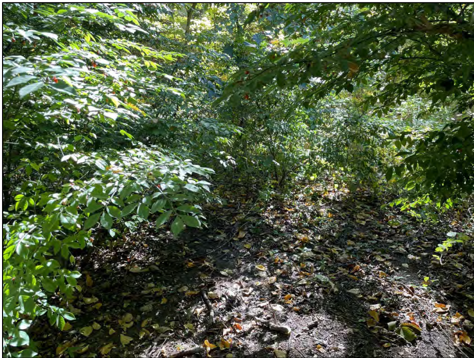
Photo No. 10.: Crest of the dam right of the spillway.
