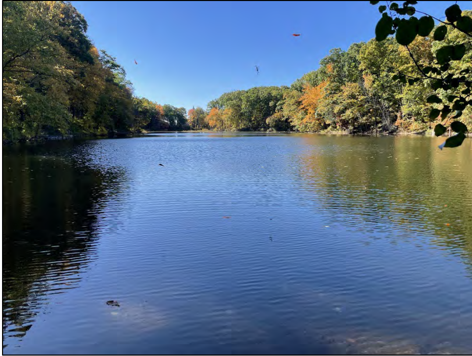
Photo No. 1.: Overview of the impoundment from near Sta. 1+50 looking upstream.
