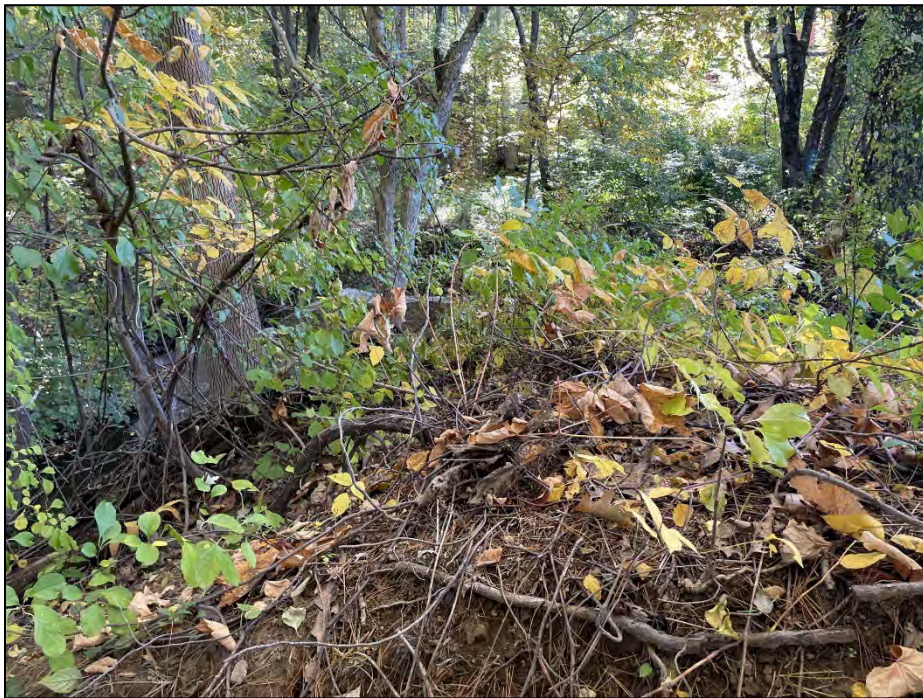
Photo No. 14.: Downstream slope from near Sta. 1+00 looking right.
