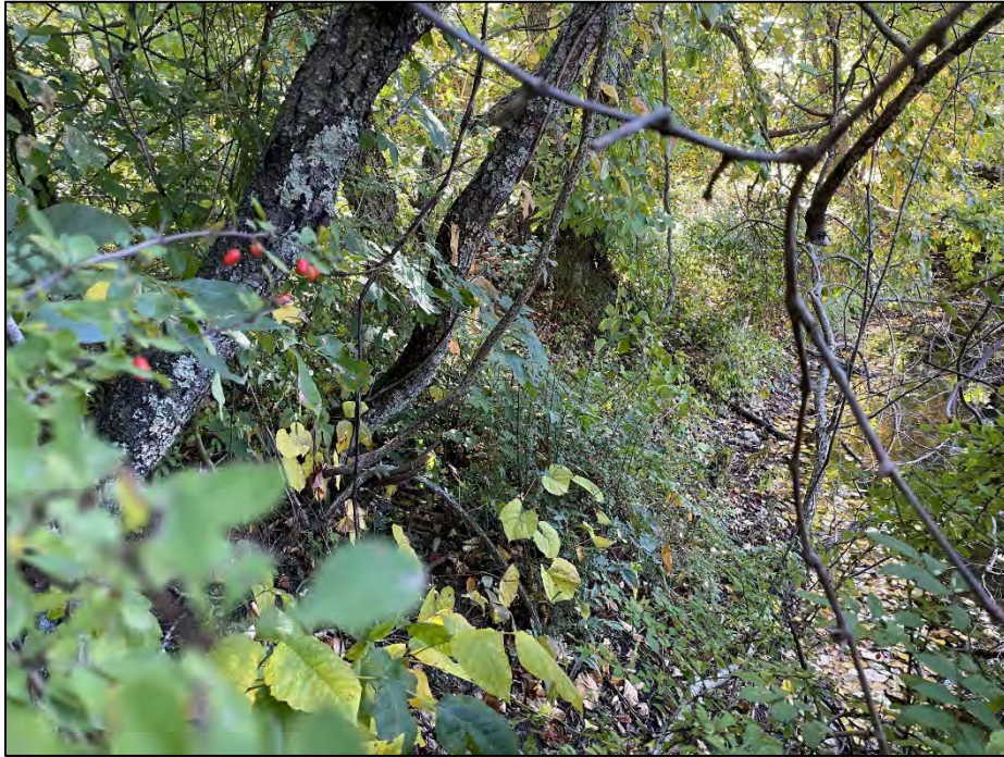
Photo No. 5.: Upstream slope of the dam right of the spillway.
