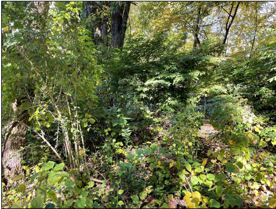
Photo No. 15.: Downstream slope right of the spillway.
