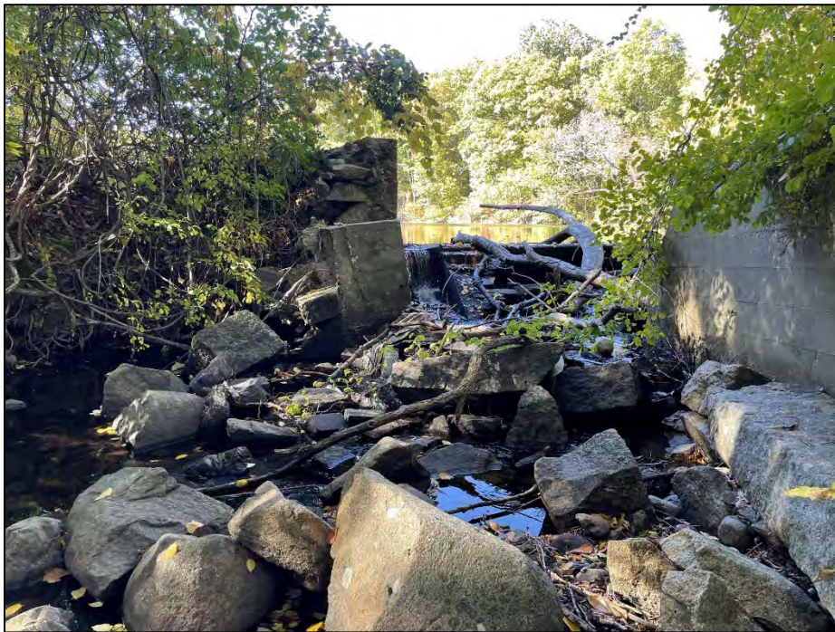
Photo No. 18.: Spillway channel from downstream channel looking upstream.
