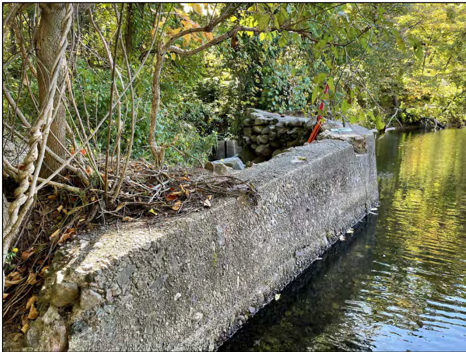
Photo No. 4.: Upstream wall from near Sta. 1+30 looking right.
